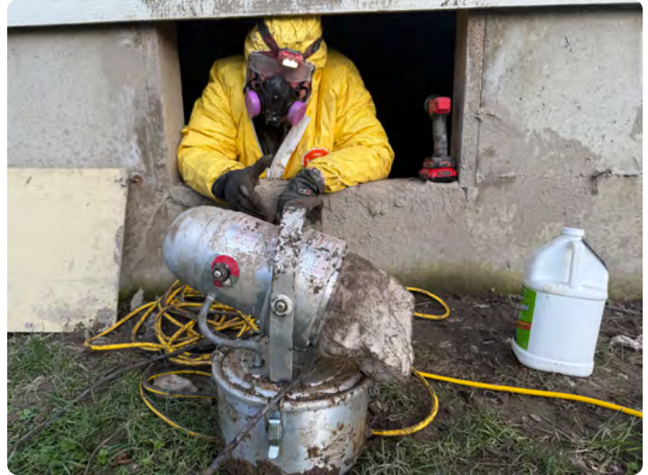
PNW ERT member Keith Skore is preparing to fog underneath a home in Sumas after the December 2025 floods. Photo by Dana Bryson.
