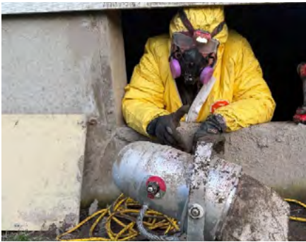
PNW ERT member Keith Skore preparing to fog underneath a home in Sumas after the December 2025 floods. Photo by Dana Bryson
